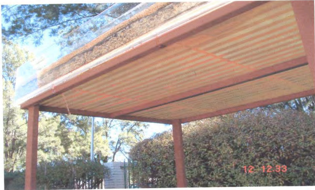
Figure 5: Drainage through the system 4,5 minutes after commencement of the test
