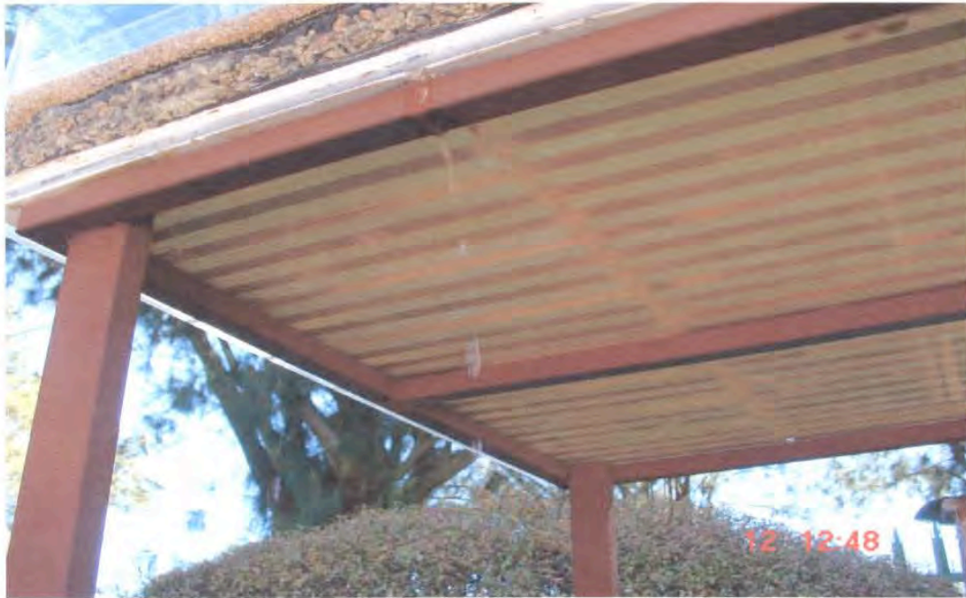
Figure 7: Thin layers of sediment deposited on the base below the channels in the board
